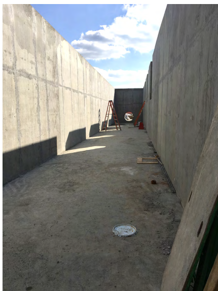
Fig 7 – A look inside the flow control channel at the Bellwood Quarry pumping station. More than 1,000 cubic yards of 5,000 psi concrete was treated with Xypex Admix C-500 crystalline waterproofing.
