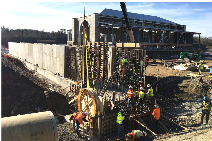
Fig 9 – Elaborate form work and reinforcement was needed to integrate multiple large pipes into the concrete channel at both the Bellwood Quarry and Hemphill pumping stations.
